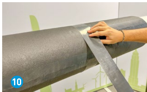
Apply ArmaFlex Ultima C tape on the circumferential seams.
