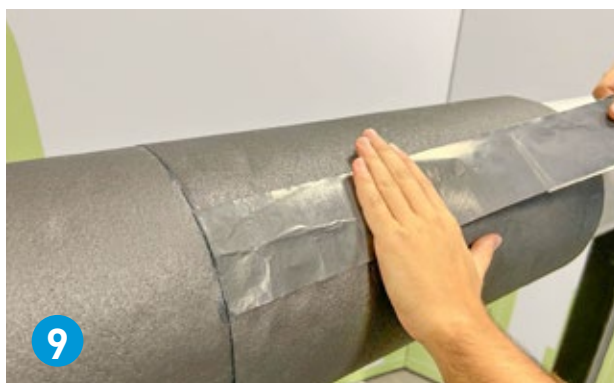
Apply ArmaFlex Ultima C tape on the longitudinal seams.
