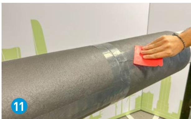
Use a plastic spatula to smooth the ArmaFlex Ultima C tape surface.
