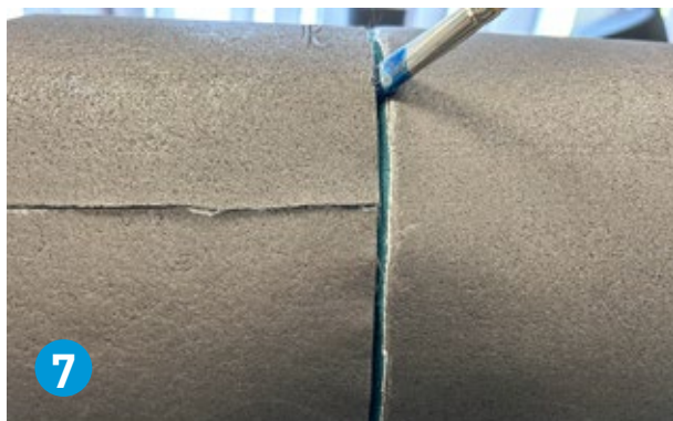
Apply adhesive onto the circumferential seams.
