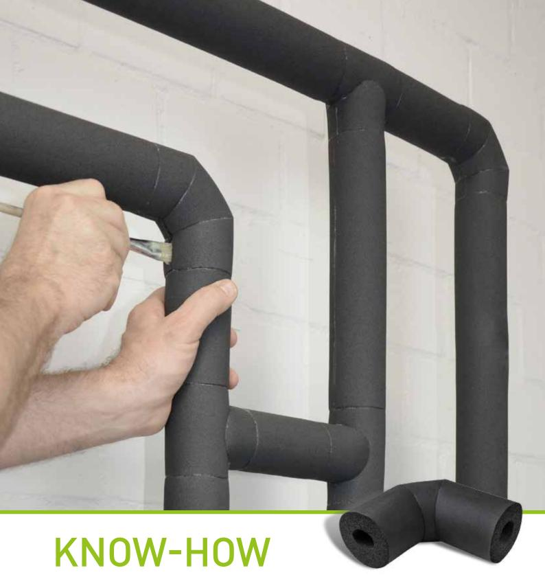
The correct installation of Armaflex on bends
