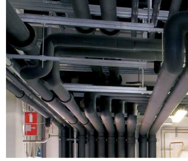
Compression in the throat of the bend can lead to a reduction in the insulation thickness and this in turn to condensation on the surface of the insulation material. If in doubt, it is best to fabricate fitting covers for bends.
